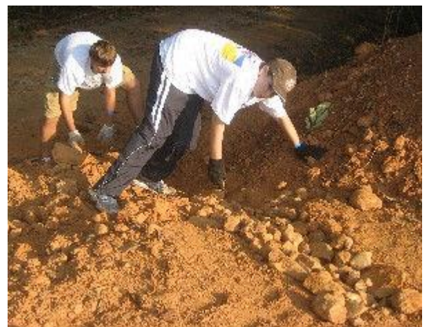
Candidates line drainage ditch with rocks.
